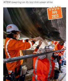
Welding the cascade shaft into place
